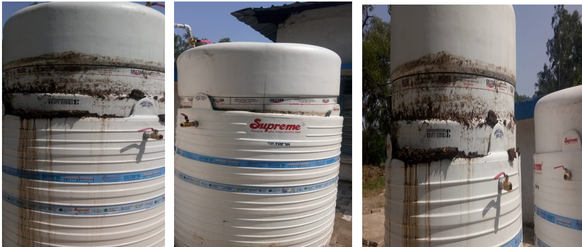
Biogas Reactors installed at 3 BRD Air Force Station, Chandigarh
