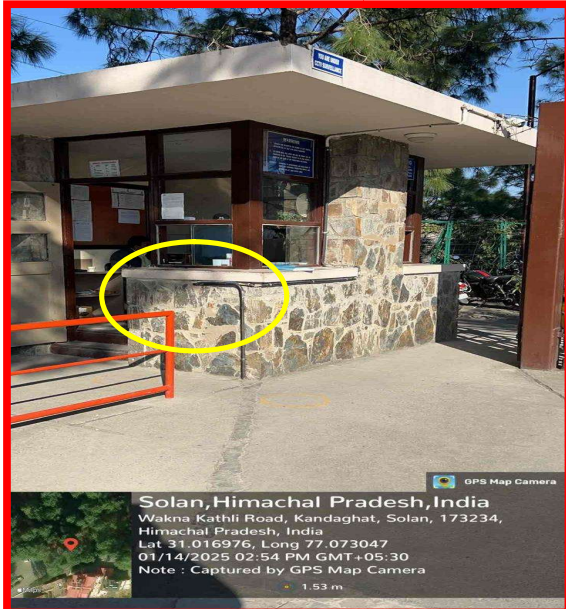
Fig: 2 Security at Main Gate JUIT with CCTV cameras installed
