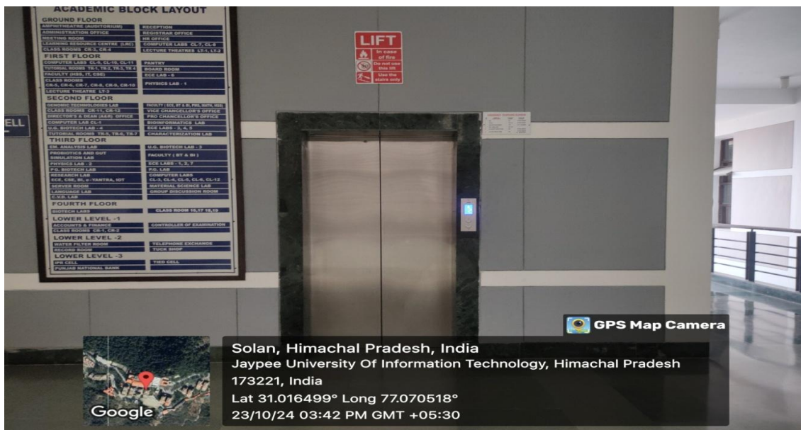
Lift facility – Image 1
